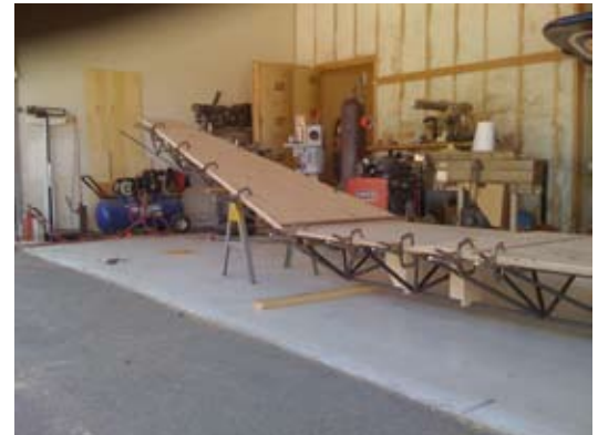
Welding without warping is a challenge on this structure.
